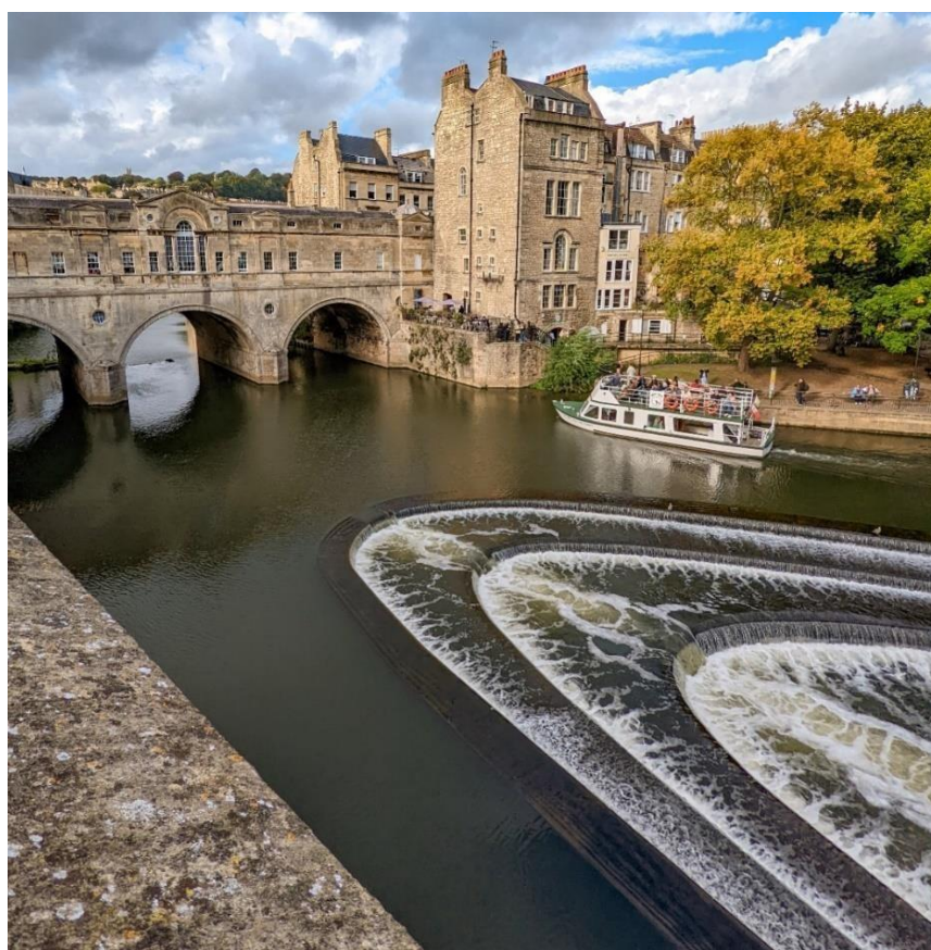
Figure 6 - Pulteney Bridge and Weir in Bath
