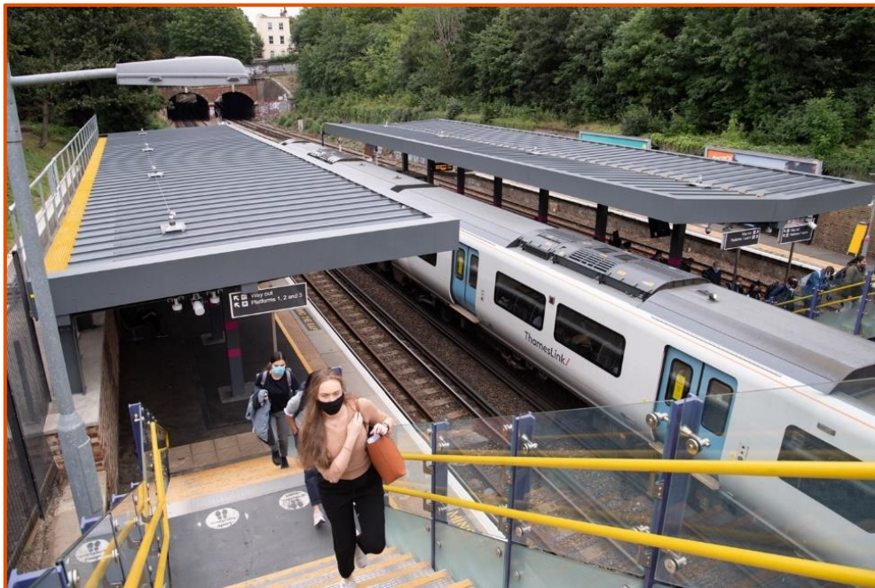
FIGURE 18: SOLAR FILM AT DENMARK HILL (SOURCE: BIPVCO)
