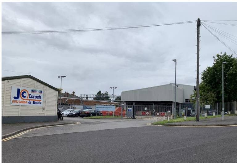
Figure 14 View of Salisbury TMD
