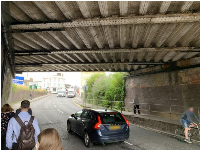
Figure 24 Walkway Beneath Fisherton Street Bridge
