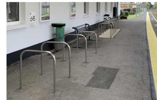
Figure 12 Sheffield Stands at Dorchester West
