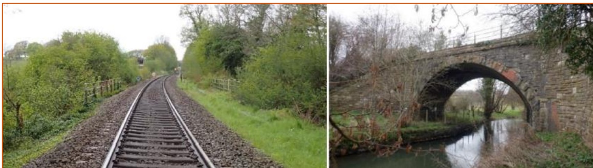
Figure 3-45: River Nadder Underbridge
