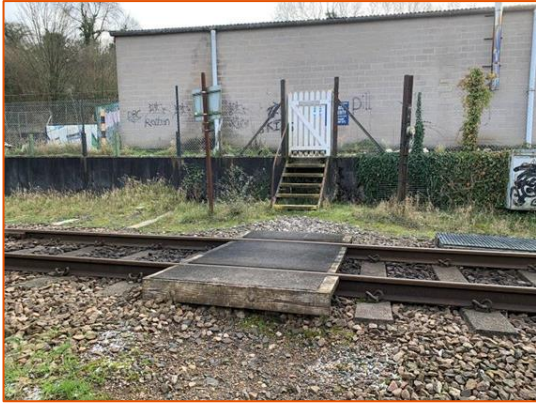
Figure 3-56: Chantry Level Crossing
