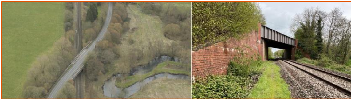
Figure 3-44: French Horn Bridge
